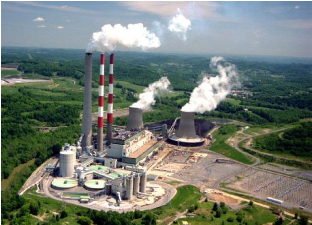
Photo courtesy of Allegheny Energy
