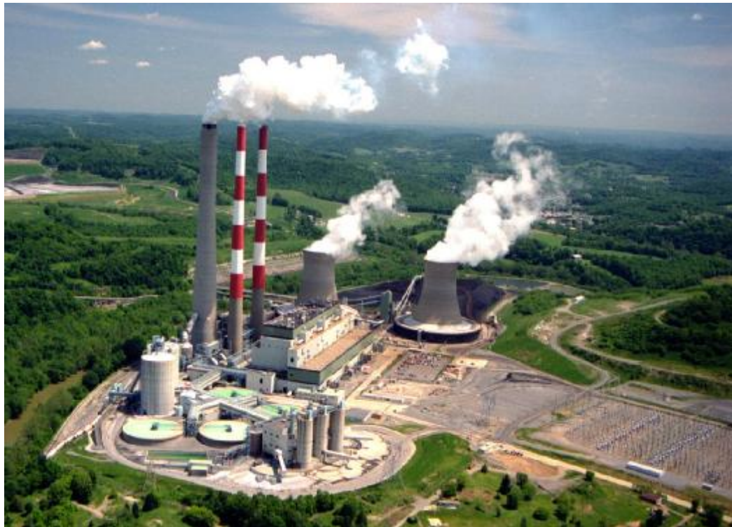
Photo courtesy of Allegheny Energy
